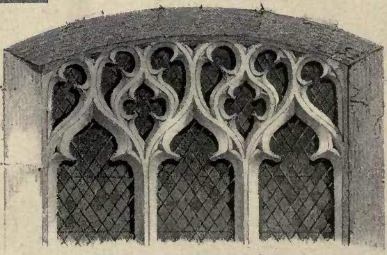
SOUTH EAST WINDOW IN AISLE.
